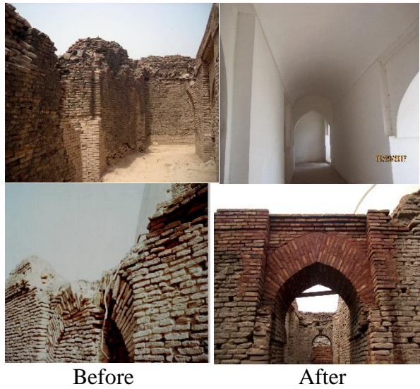
Figures 10: Vault roofs and walls of attached verandah, Old and Present
