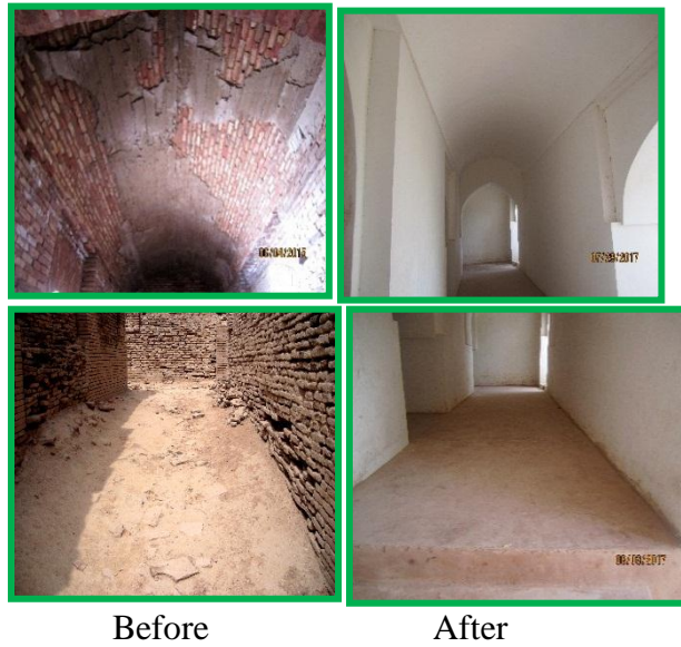
Figure 12: Use of Kankar lime plaster, repairing of interior walls and vaults
