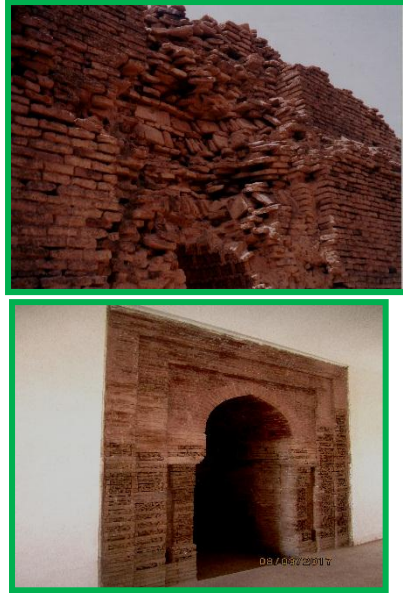
Figure 22: Repairing of mehrib, the tiles were re-fixed and calligraphic work was completed under the principles of conservation.
