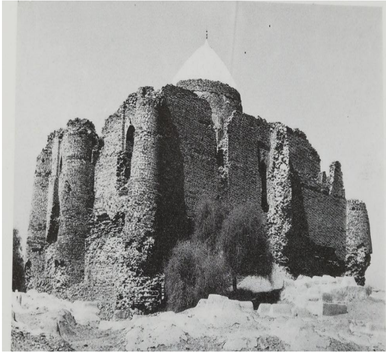
Figure 2: Tomb of Khaliq Wali before repairing with complete condition of central hemispherical dome.
