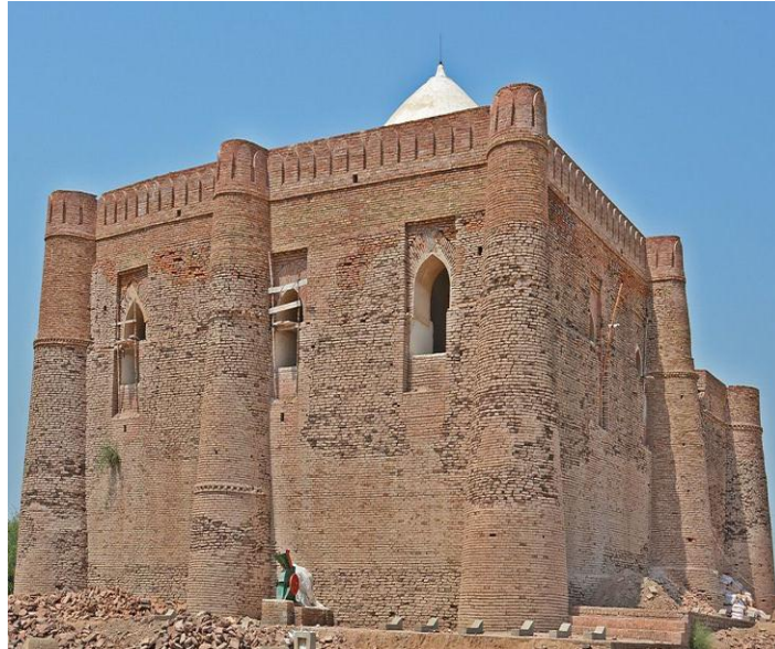
Figure 4: The image shows the height, rectangular plan and Citadel of the tomb which indicates the concept of military architecture
